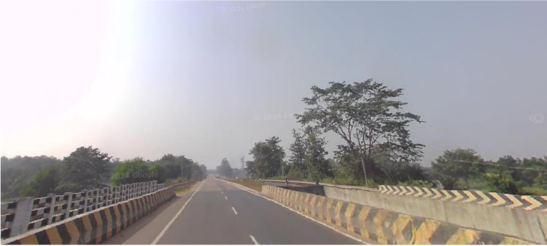
IMAGE: BRIDGE ; RISKLEVEL: MEDIUM ; COORDINATES: 21.9698064, 86.7174948 (60.9Km)
